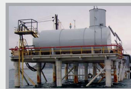
Exhaust incineration of gasoline vapours
